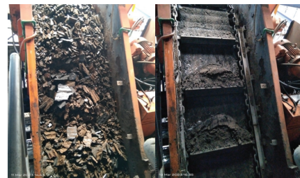
CoalTreat's impact on furnace slagging can be seen as waterwall and pendant slag shedding is observed within the first day of treatment. After a week of continuous treatment, the finer, friable consistency of treated bottom ash is observed.
